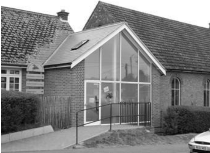
A Vision Achieved! The New Side Entrance.
